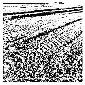
Figure 2-43. Airstrip - Surface Grading
