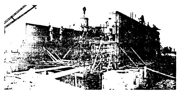
Figure 2-122. Station 1341 - Pouring Side Walls
