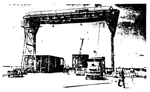
Fi: r= 2-231. 25 Ton Gantry Crane - Barge Slip - Assembly Area - Site Elmer
