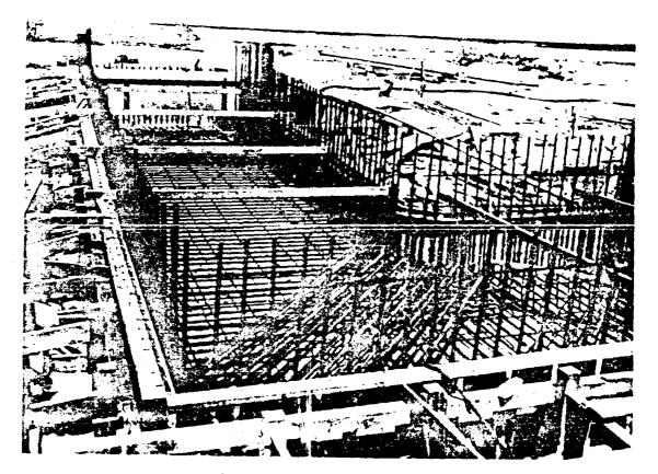
Figure 2-146. Station 2200 - Co.ner Repforcement
