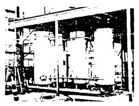
Figure 2-85. Station 60 - Air Receivers Installed 2-83 shows the west wall of Station 60. The Station was estimated 66% completed as of 8 December. Figure 2-84 shows Station 60 and area compound looking from the ocean towards the lagoon. Figure 2-85 notes the air receivers installed in Station 60.
