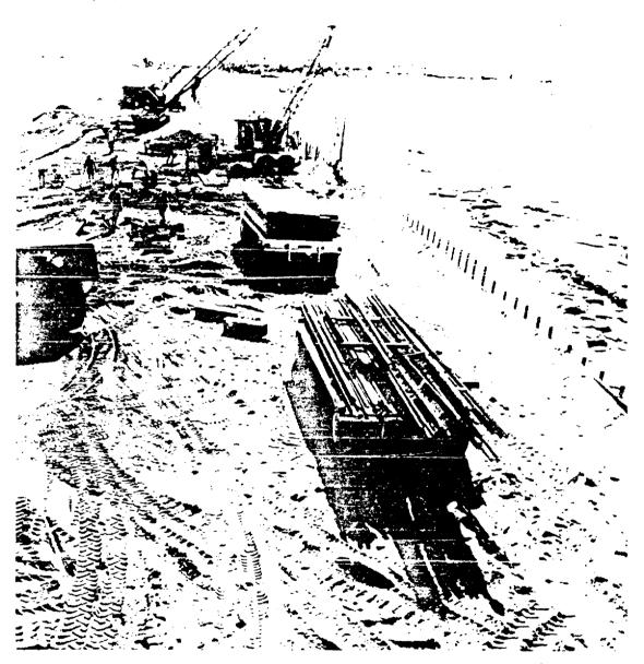
Figure 2-210. Charlie Causeway - Construction of Bulkhead
