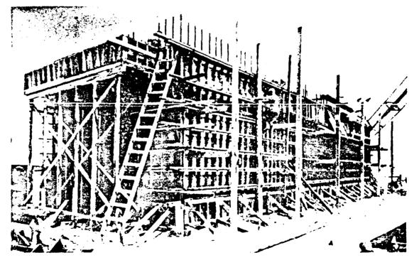
Figure 2-137. Statron 1550 - Construction of Wall Forms
