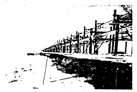
Figure 2 213. Charlie Causeway - Erosion from Wave Action
