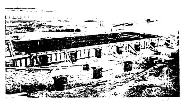
Figure 2-2. Typical H-pile Foundation
