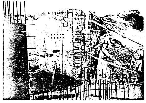
Figure 2-149. Station 2201 - Bonding to Old Structure
