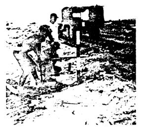
Figure 2-15. Measuring Chaining Bucks
