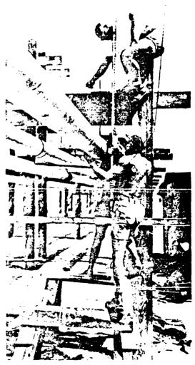
Figure 2-16. Vertical Alignment of Pipe Arrays
