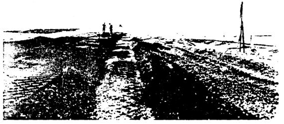
Figure 2-222. Ruby to Sally Causeway - Primary Grading
