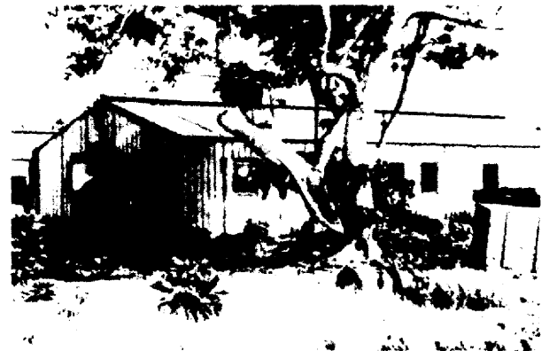
Figure 2-186. Operations Building - Rongerik
