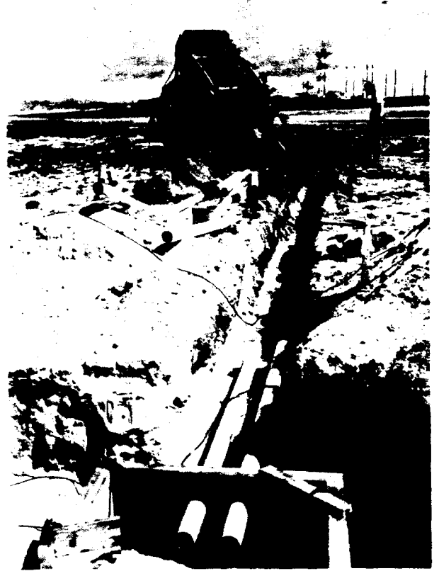
Figure 2-191. Excavating for Conduit from Runway
