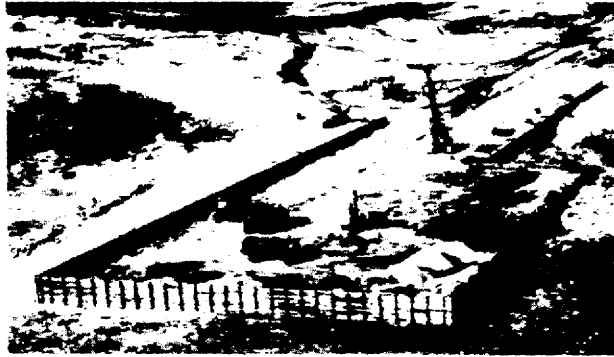
Figure 2-156. Bulkhead Construction - Sally
