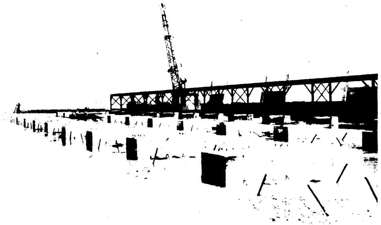
Figure 2-87. Station 1524 - First Row of Steel Pipe Supports Erected
