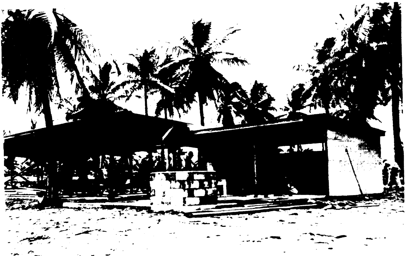
Figure 2-176. TG 7.3 Recreation Facilities - 80% Complete
