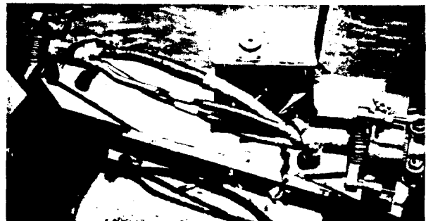
Figure 2-166. Cable Being Spliced
