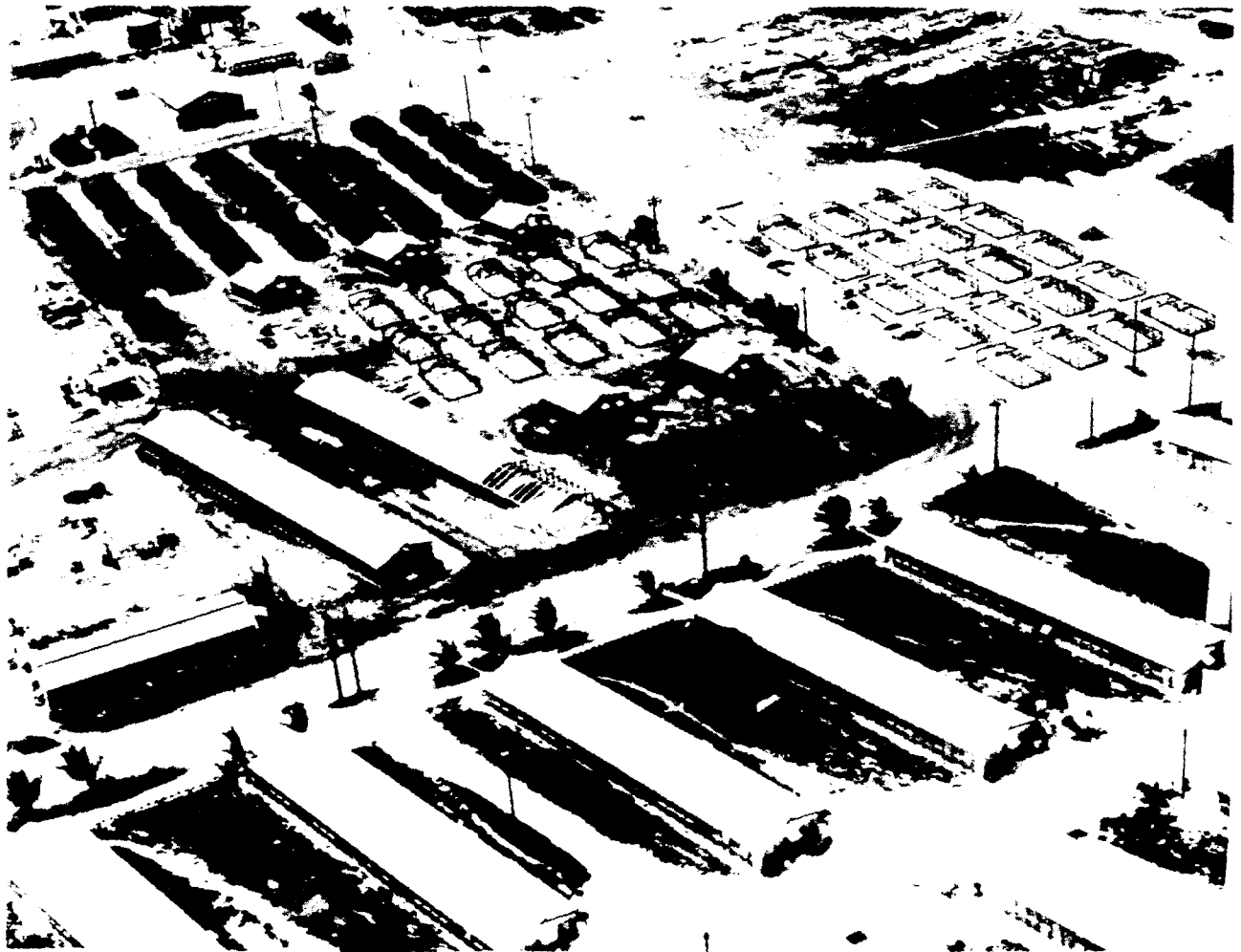
Figure 2-198. New Housing Area - Elmer - 85% Complete
