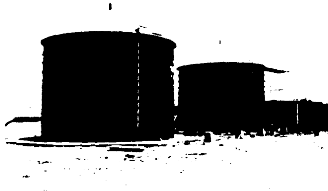
Figure 4-23. Redwood Stave Fresh Water Storage Tanks
