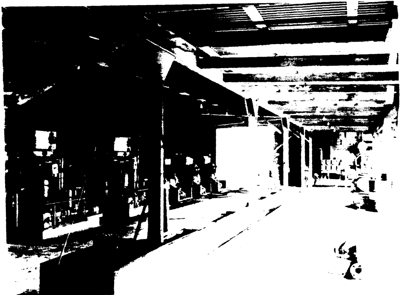
Figure 4-19. Distillation Plant - Nan
