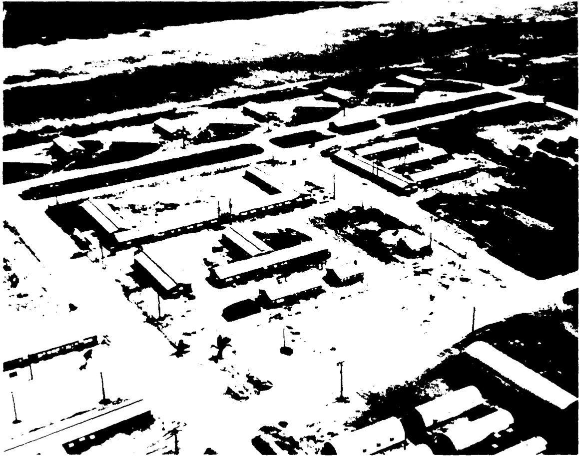
Aerial View, Parry Island, Showing Quonsets, Administrative Area Security Compound, and Personnel Barracks
