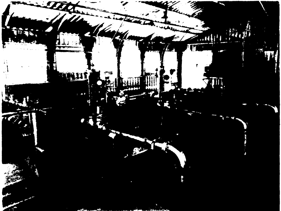
Parry Island: Interior of Salt Water Pump House
