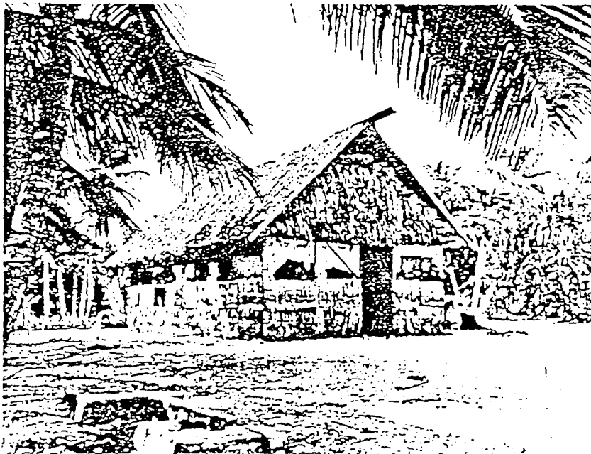
FIGURE 1.1—Typical construction of the Marshallese homes to illustrate the exposure environment of the Marshallese and the lack of shielding from gamma radiation.
