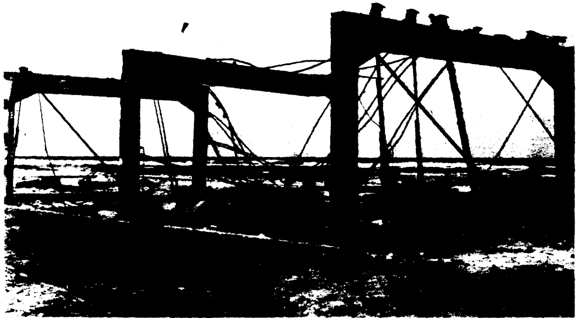
Job 5 Support & Roll-up Program Incuded Disposal of Damaged Structures Such as This Station 3.3.8.
