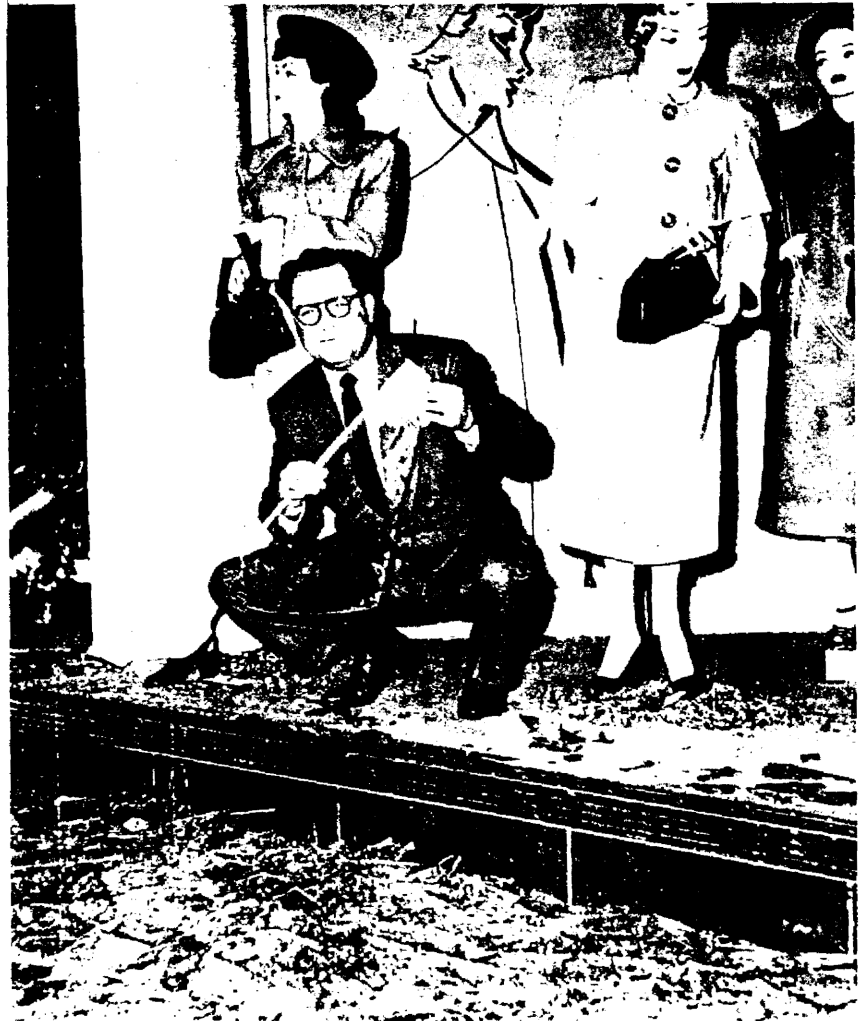
FIGURE 7. — A downtown Las Vegas window, showing how the glass was sucked out by the rarefaction wave, rather than pushed in by the compression wave resulting from the November 1, 1951, nuclear test at the Nevada Test Site.
