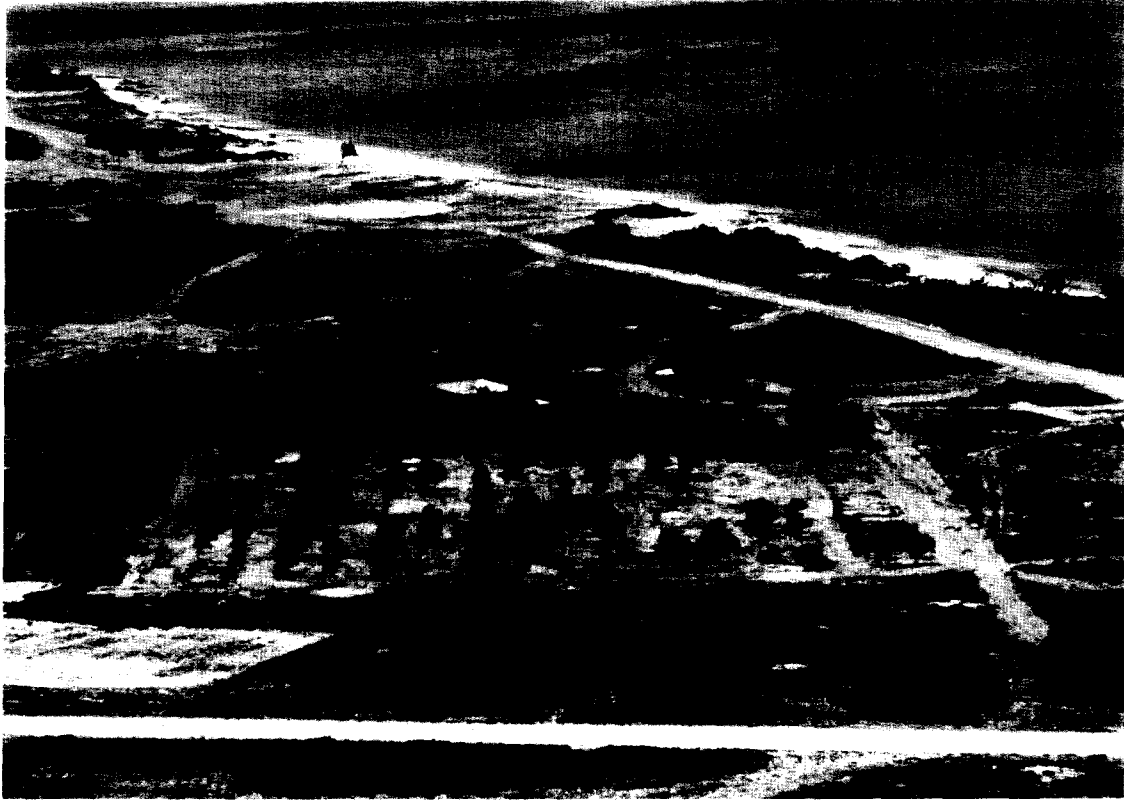
FIGURE 6-28. LLL RESEARCH AREA ON ISLAND JANET. The "farm" viewed from the northwest at the completion of cleanup. Surface soil was removed from the area at lower left, just outside the farm area. (Summer 1979)
