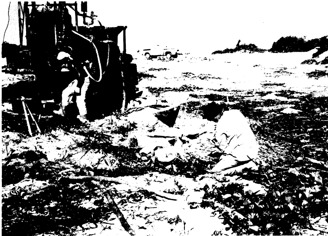
FIGURE 6-9. CORING DRILL AT THE AOMON CRYPT. The center monument area as viewed toward the west during drilling operations. (January 1979)
