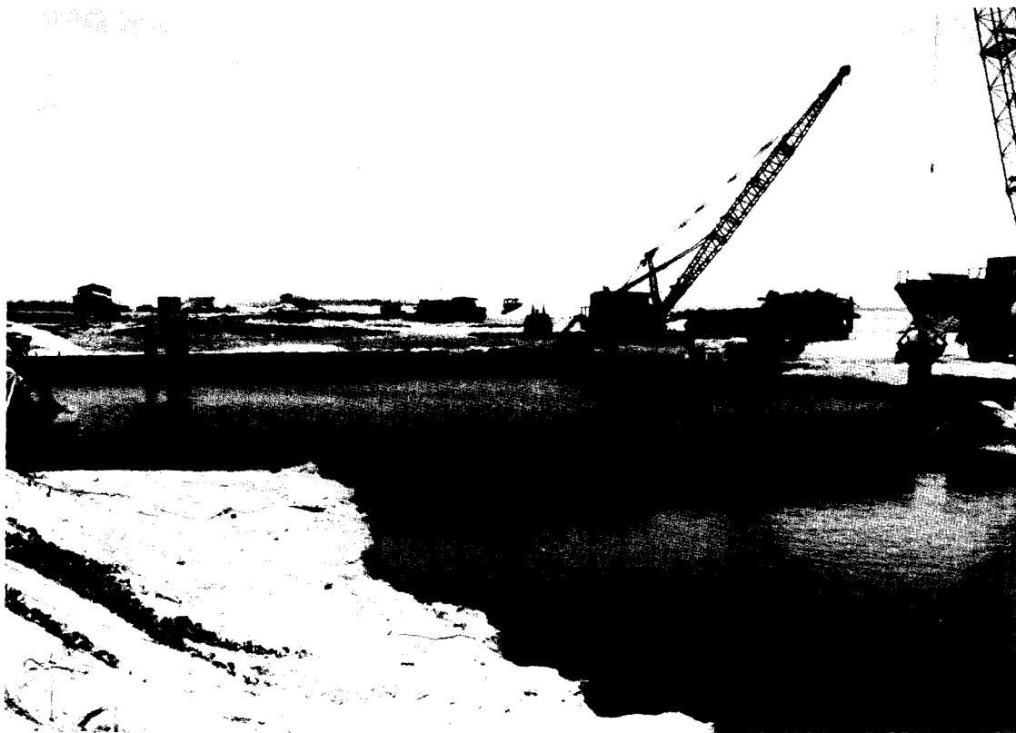
FIGURE 6-15. AOMON CRYPT JUST BEFORE BACKFILLING. All excavation completed, the pool is ready for backfill. (May 1979)
