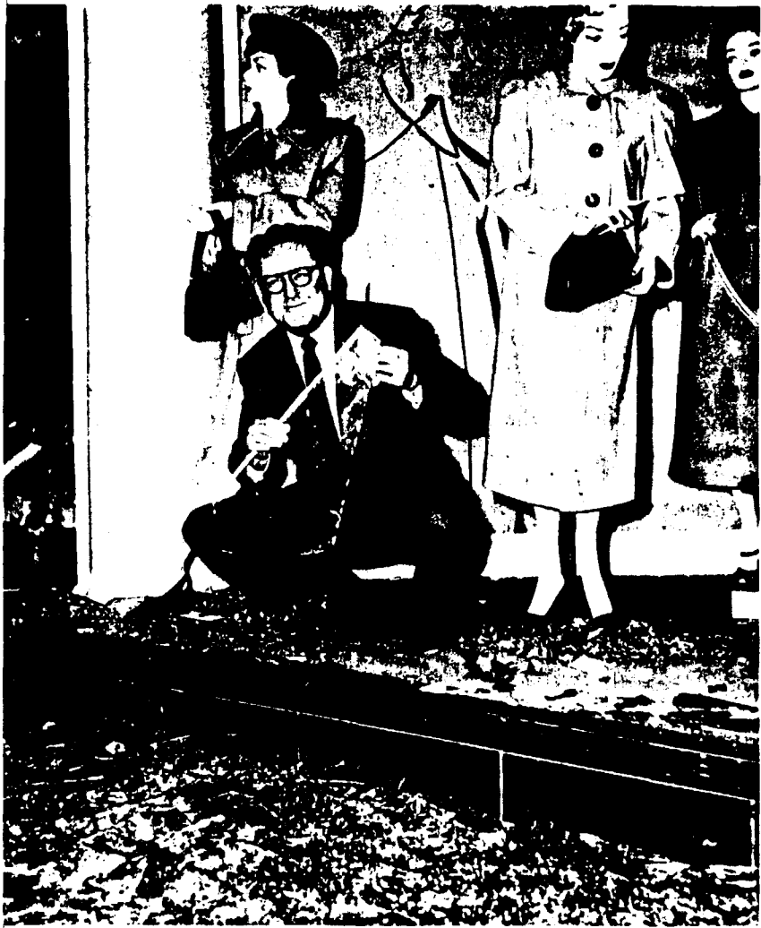
FIGURE 7.—A downtown Las Vegas window, showing how the glass was sucked out by the rarefaction wave, rather than pushed in by the compression wave resulting from the November 1, 1951, nuclear test at the Nevada Test Site.
