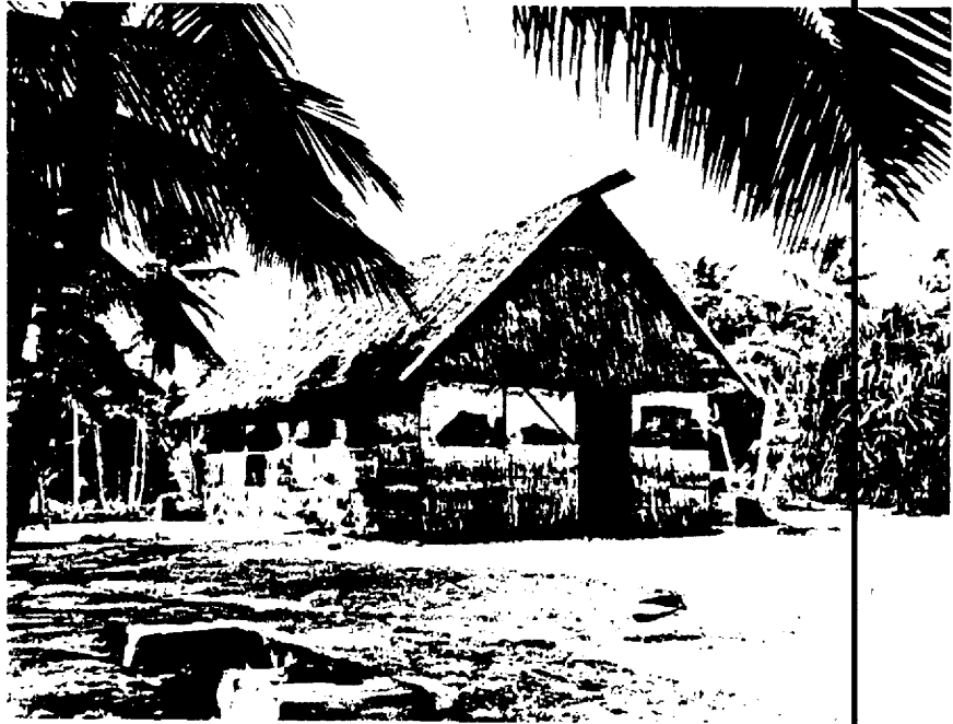
FIGURE 1.1— Typical construction of the Marshallese homes to illustrate the exposure environment of the Marshallese and the lack of shielding from gamma radiation.
