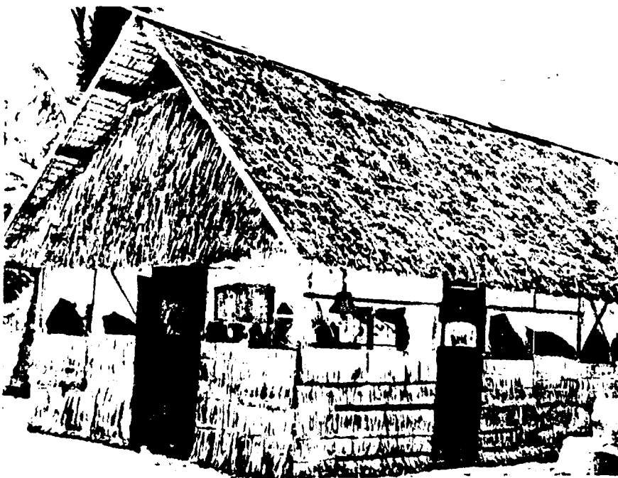
F.g. 1.1 The Living Area on Rongelap Island, Indicating the Light, Open-type of Construction
