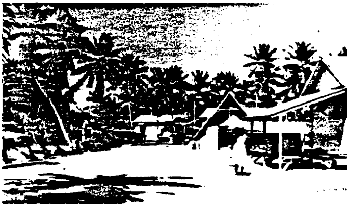
Rebuilt village on Rongelap to which people returned in 1957.
