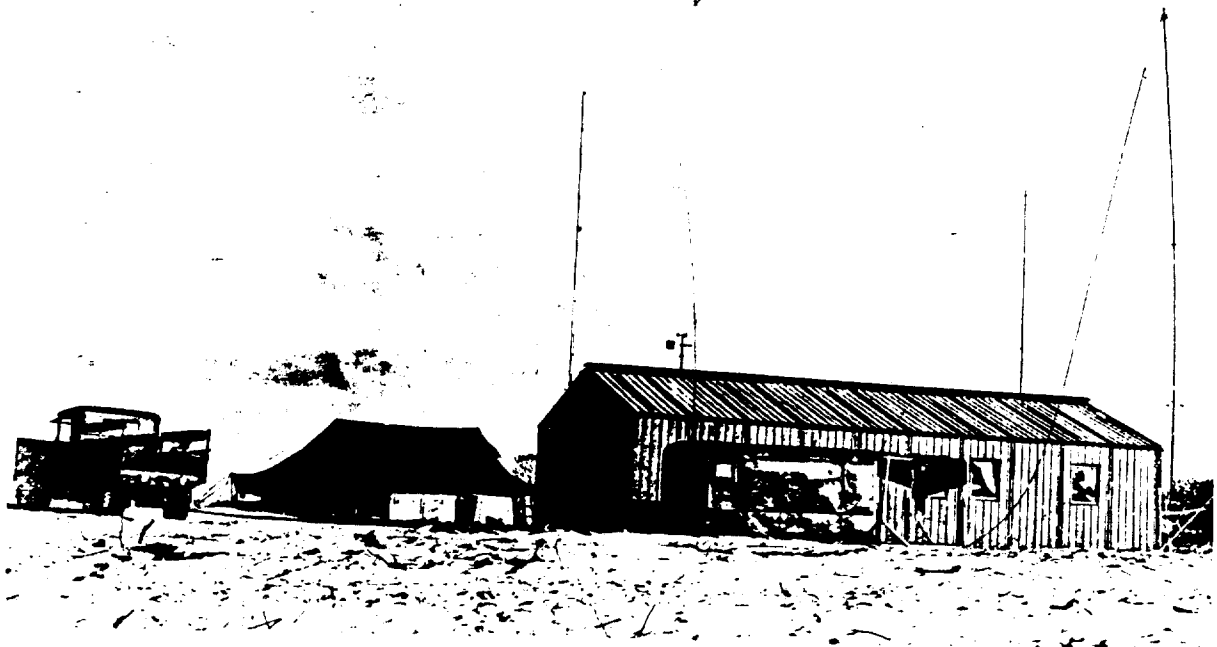
Figure 64. Photo of Rongerik installation, CASTLE.
