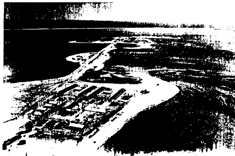
FIGURE 1-44. CONSTRUCTION CAMP ON LIDILBUT (GENE) ISLAND.
