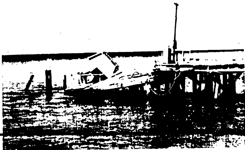
FIGURE 3-2. DELAPIDATED BOAT DOCK.
