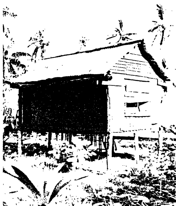
COPRA DRYING SHED — RAISED ON SUPPORTS
