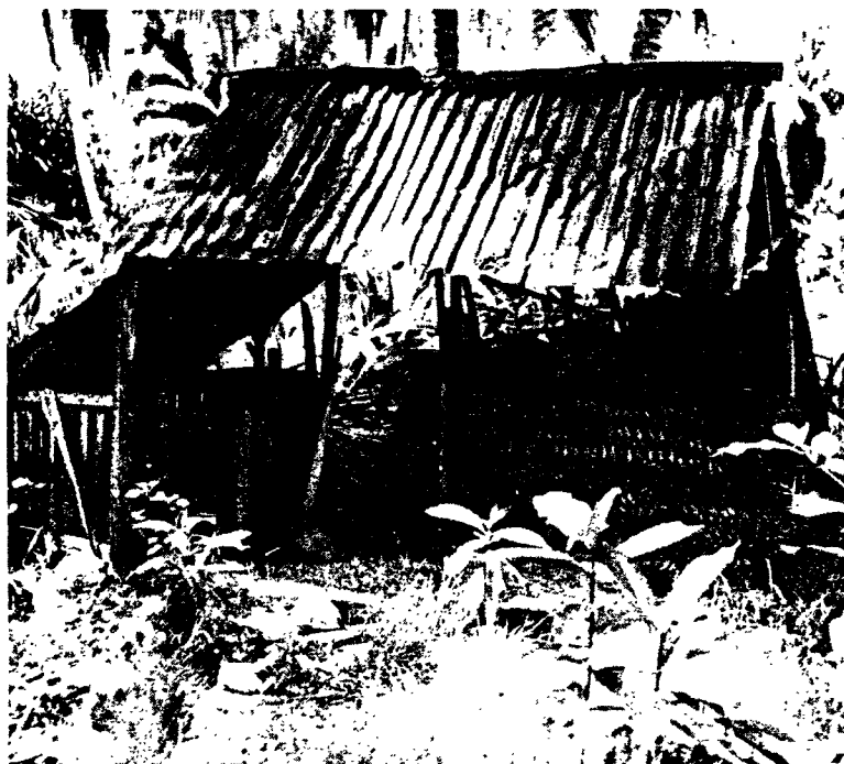
DRYING SHED — GROUND LEVEL
