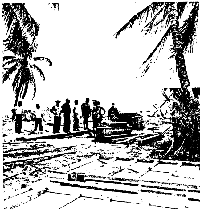
NATIVE COUNCIL INSPECTING CONSTRUCTION
