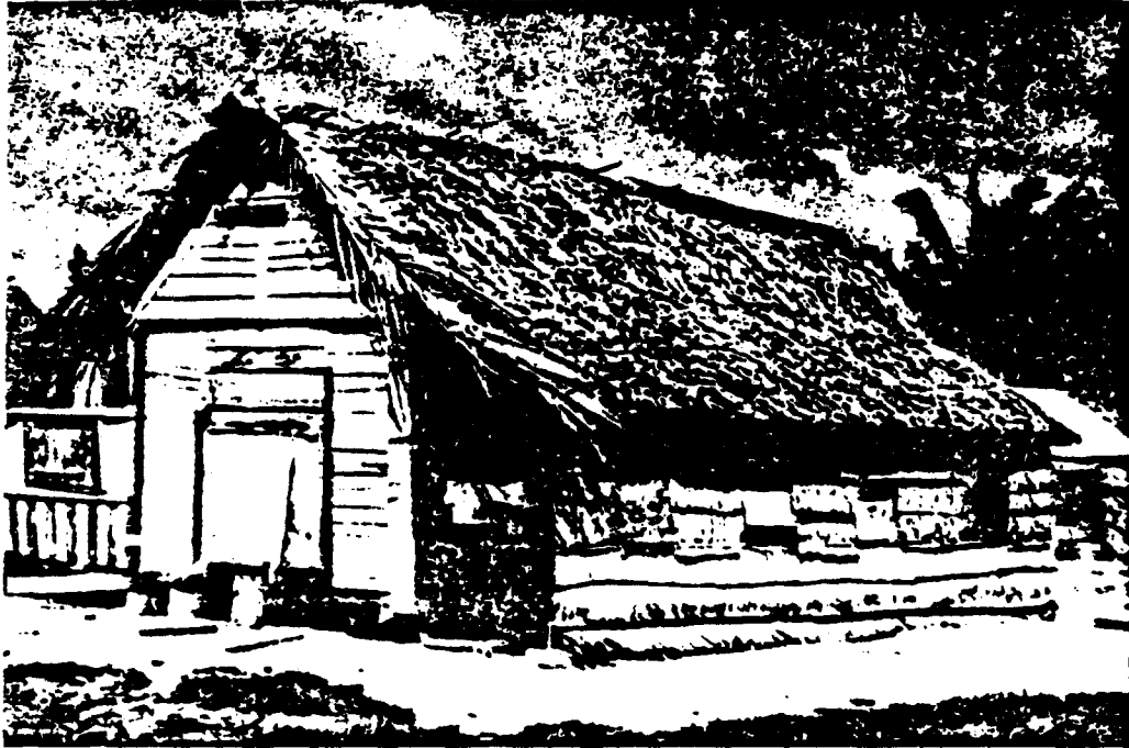
Figure 2.4 House partially constructed of lumber.
