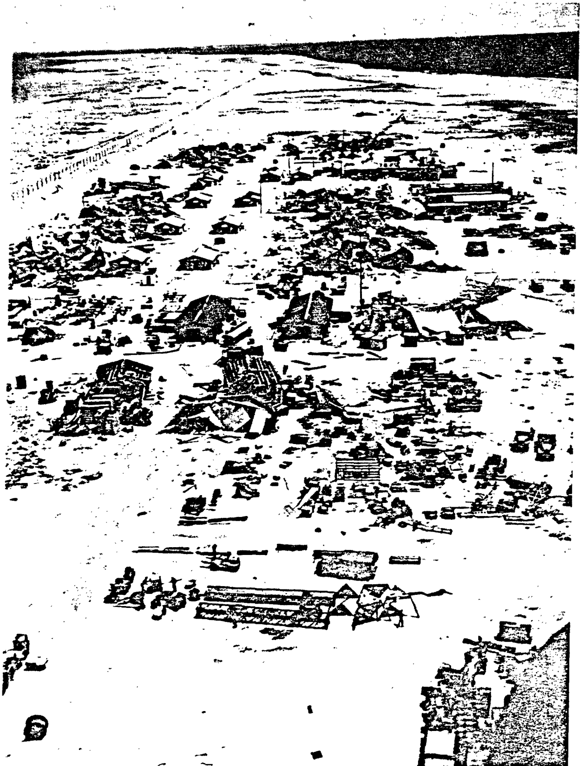
Post SHOT! Damage, Eninman Island, Bikini Atoll
