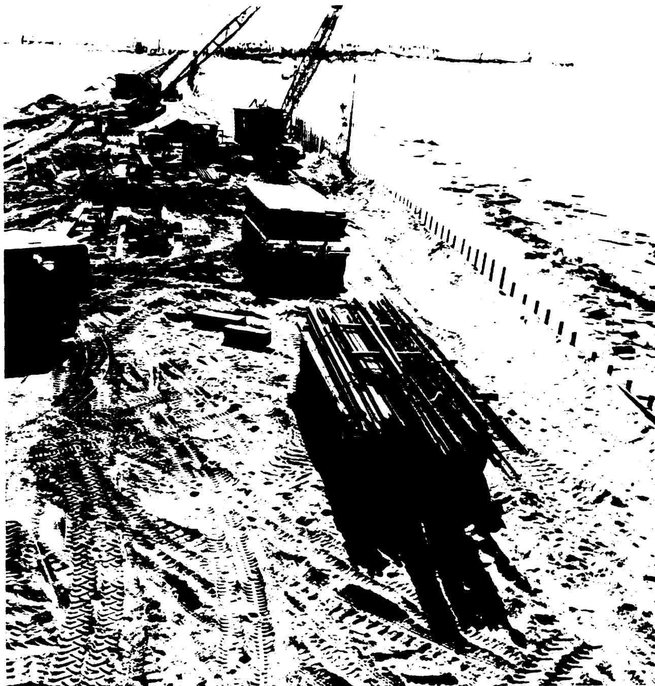
Figure 2-210. Charlie Causeway - Construction of Bulkhead
