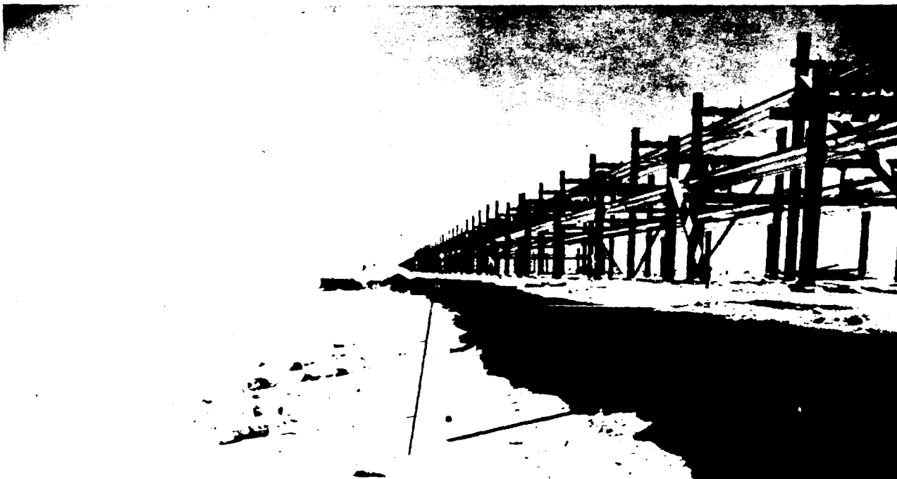
Figure 2-213. Charlie Causeway - Erosion from Wave Action
