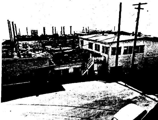
Fig. 1. The original wooden D Building which housed the chemists and metallurgists in CMR Division. Note that the chemical hoods of the laboratories on the first floor were vented individually, usually without filtration.
