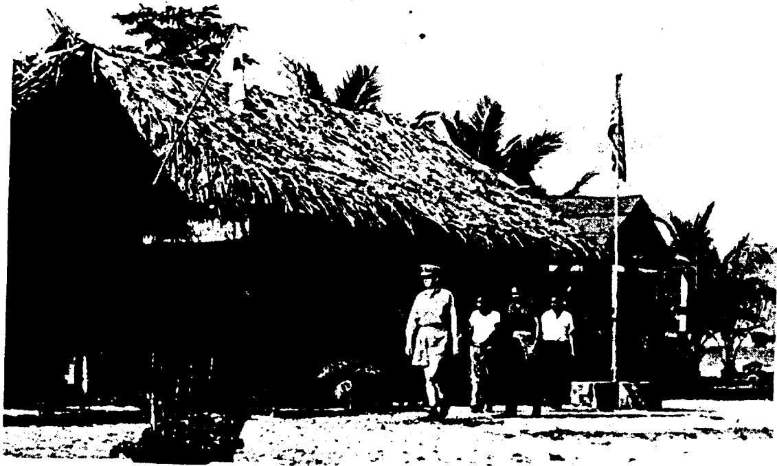
School house and adjacent di spensary on Satawan
