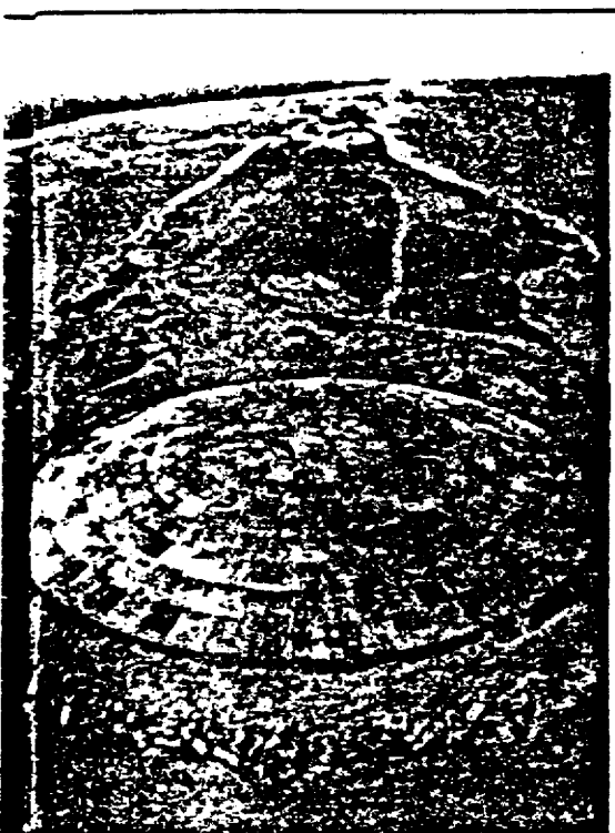
(left) People walking on the concrete dome covering an atomic bomb crater on Runit Island, Enewetak atoll. (below) Nuclear clean up on Runit Island. (left) U.S. Army personnel in full protective gear. (right) Army personnel mixing plutonium-contaminated soil with cement to form the massive concrete dome.
