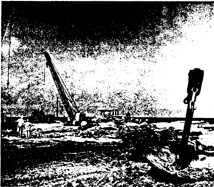
Cranes are used to pick up and load heavy metal debris at the dock area on Enyu Island during cleanup operations.
