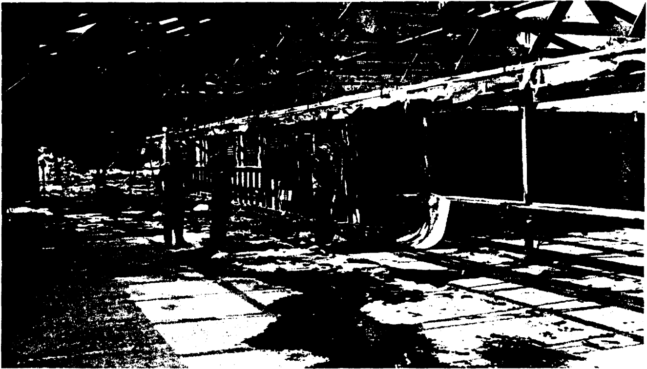
Admiral Mustin, Colonel Rawlings and Ogle inspect the mess hall on Bikini Island. Building is in relatively good condition except that it lacks roof covering.
