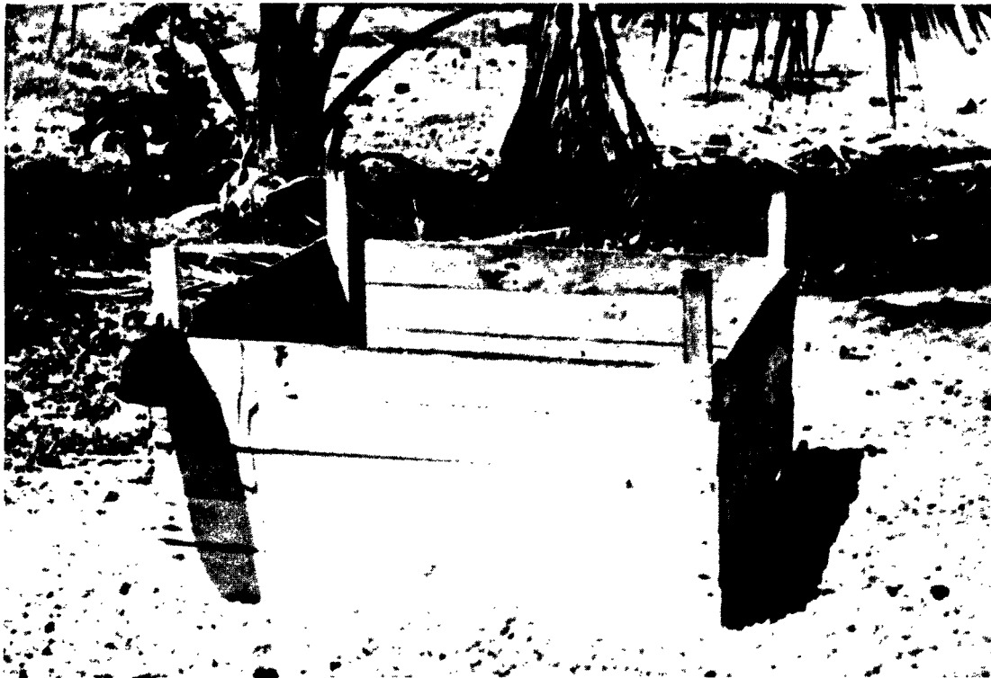
Figure 2.7 Well (No. 22 on Figure 2.1). This well was approximately 2-by-2-ft square and 12 ft deep. The sides were cased with coral masonry.
