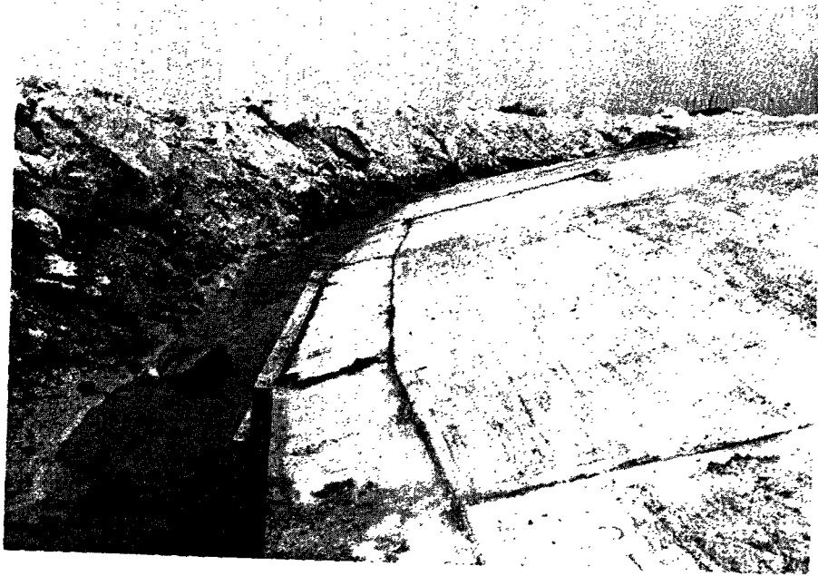
FIGURE 8-43. KEYWALL EXPANSION JOINT.
