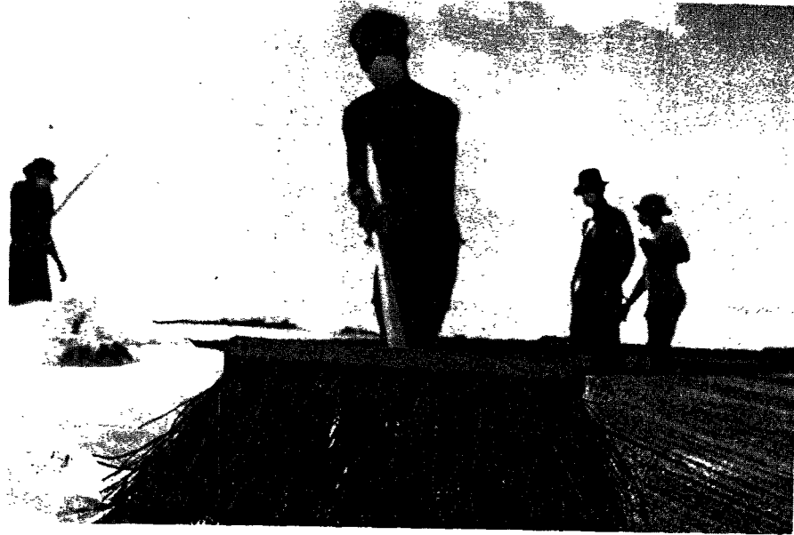
FIGURE 8-48. BROOM-FINISHING A CAP SECTION.
