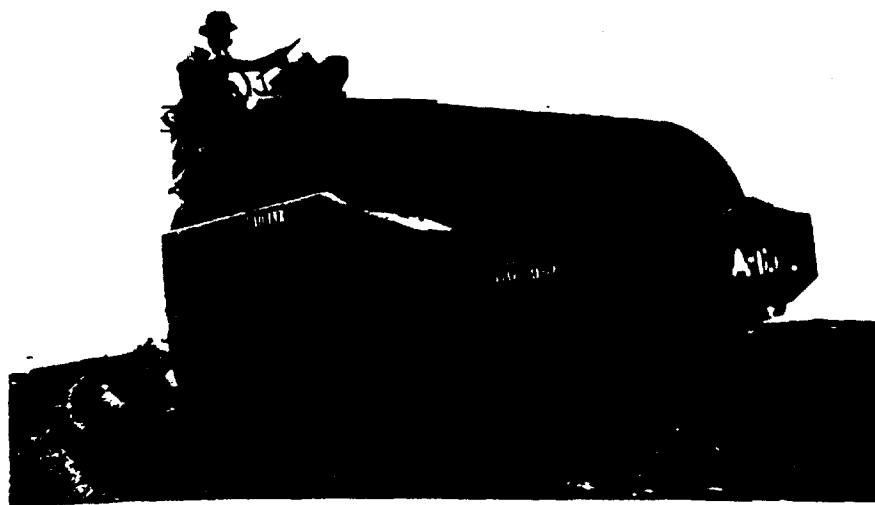
FIGURE 8-33. COMPACTING SOIL-CEMENT MIXTURE.
