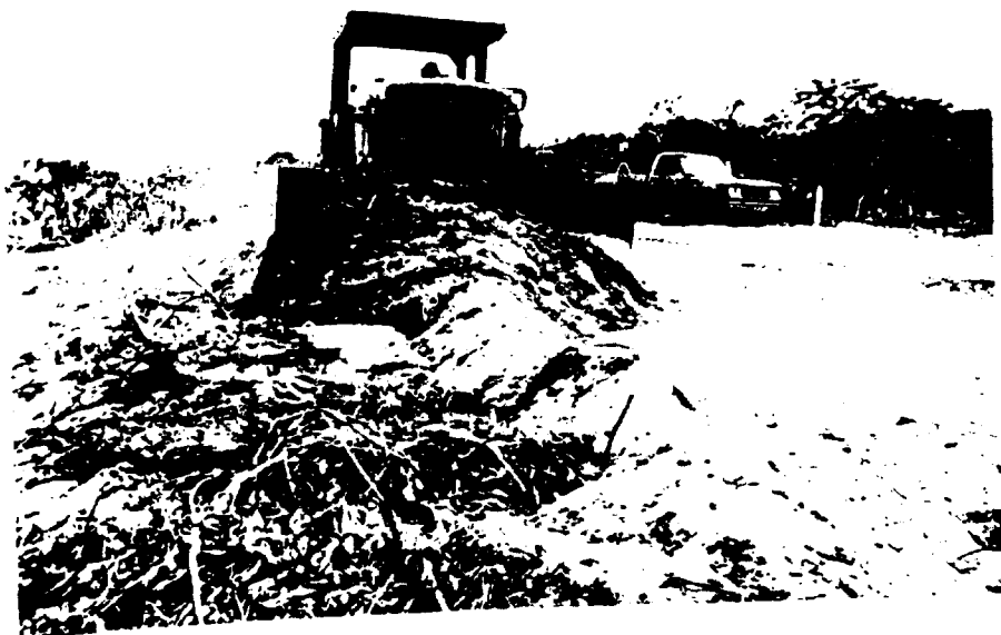
FIGURE 6-4. SOIL REMOVAL USING D8K DOZER.
