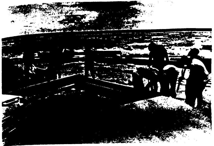
FIGURE 8-45. WOODEN CAP FORMS WITH TAPERED KEY.
