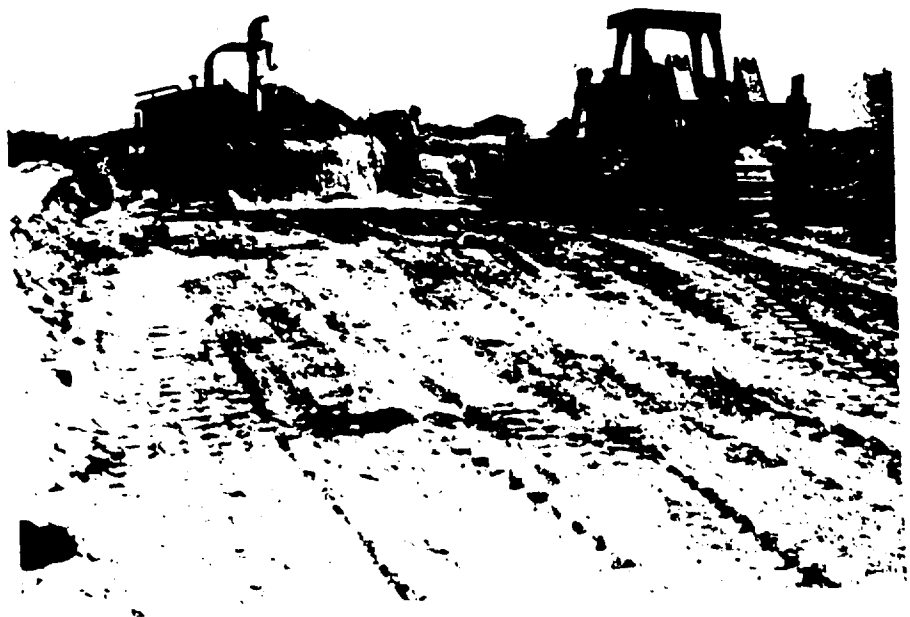
FIGURE 6-6. BACKBLADING OPERATION.
