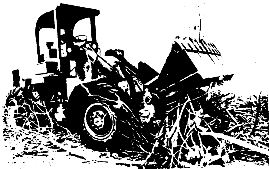
FIGURE 6-5. BRUSH REMOVAL USING FRONT LOADER.
