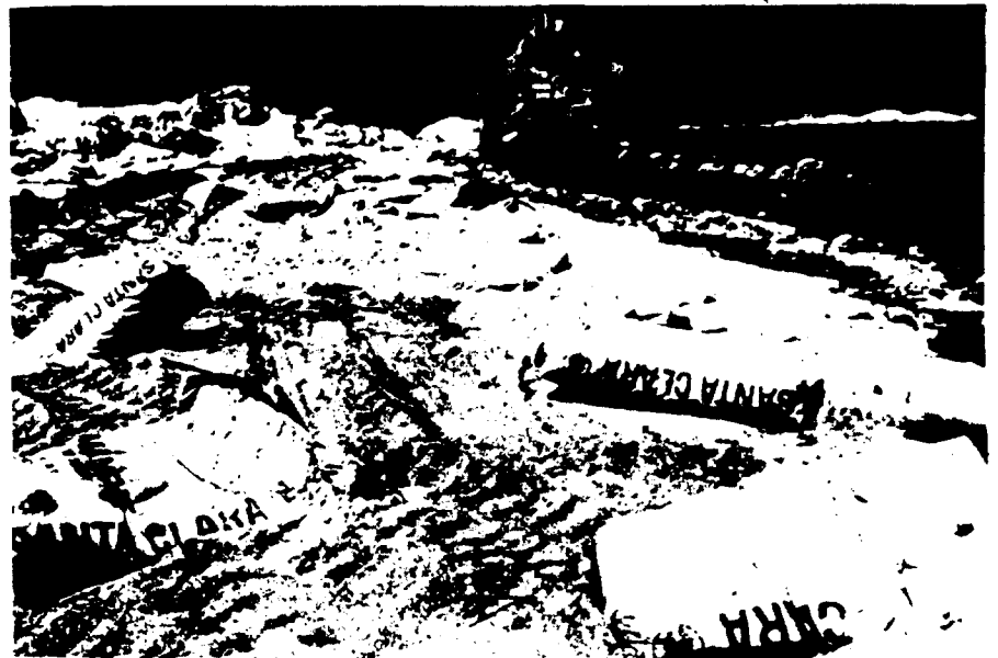
FIGURE 8-30. CEMENT BAGS PLACED FOR SOIL-CEMENT MIX.
