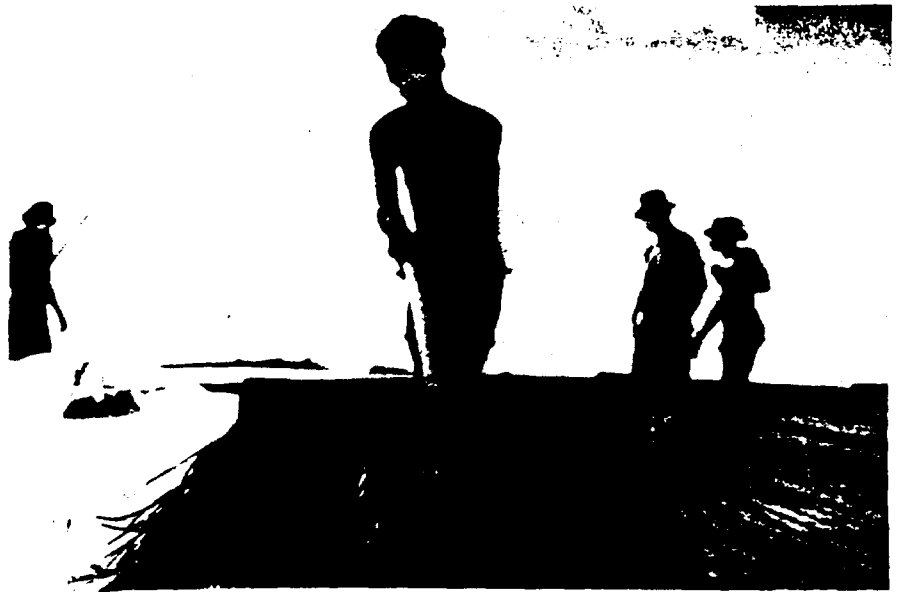
FIGURE 8-48. BROOM-FINISHING A CAP SECTION.
