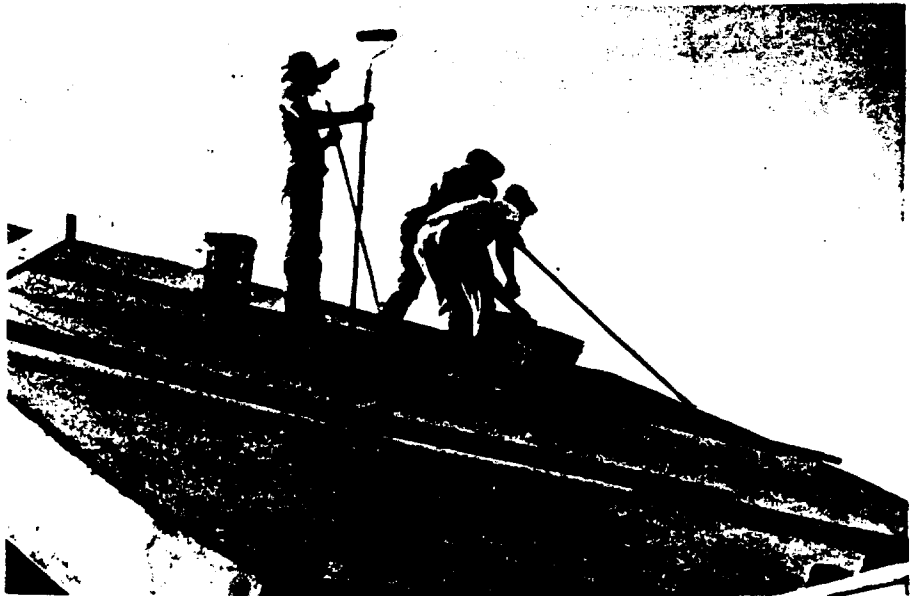
FIGURE 10-18. PAINTING THE ROOF.
