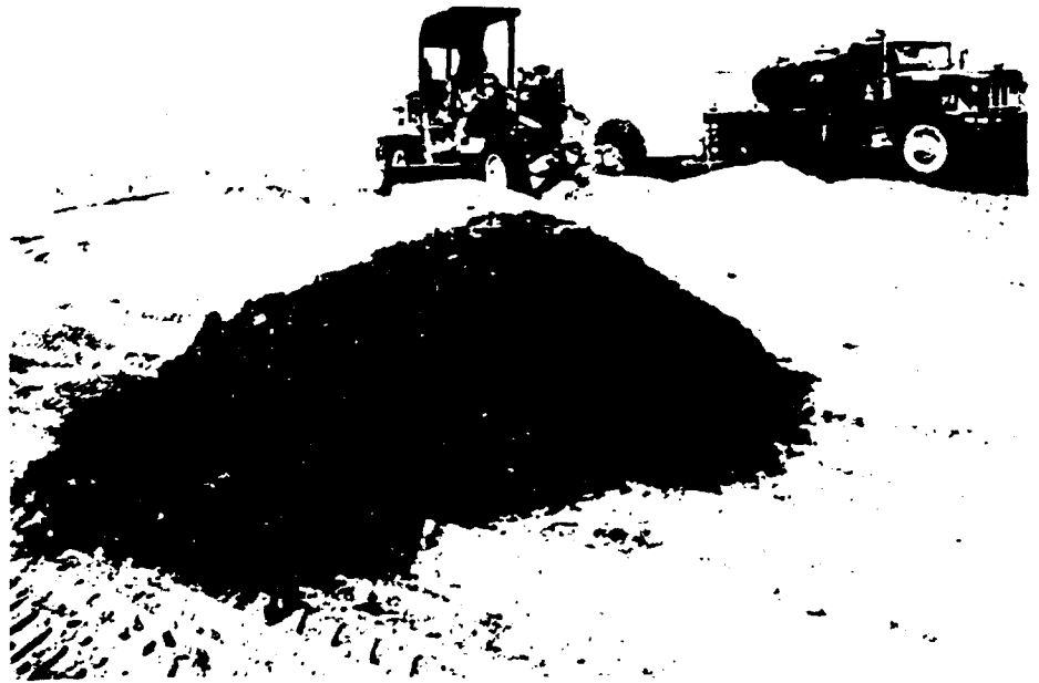
FIGURE 8-29. SPREADING SOIL WITH A GRADER.
