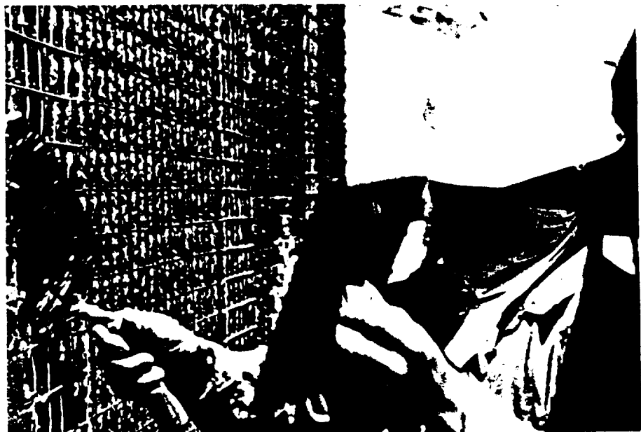
FIGURE 10-16. APPLYING CEMENT PLASTER.
