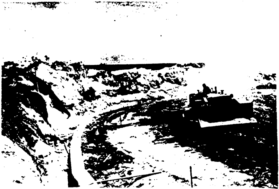
FIGURE 8-31. MIXING SOIL AND CEMENT WITH DISC HARROW.
